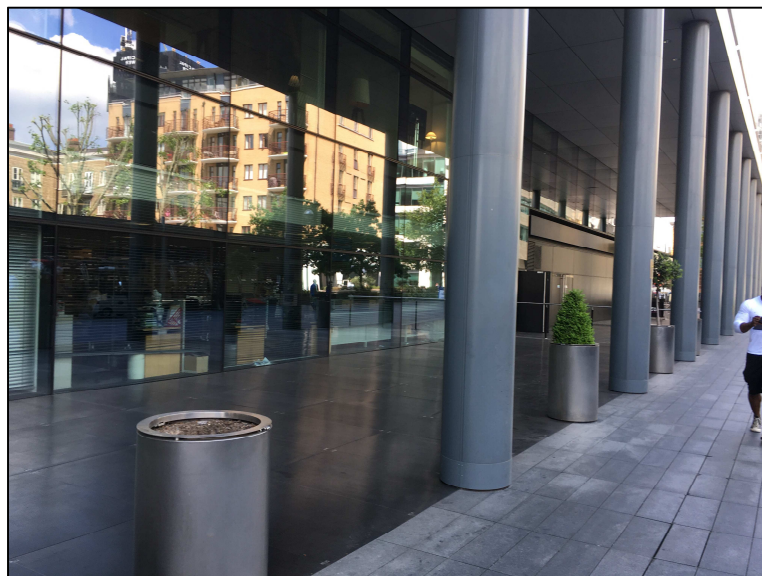
Figure 1.4: Existing Lamb Street (south)
