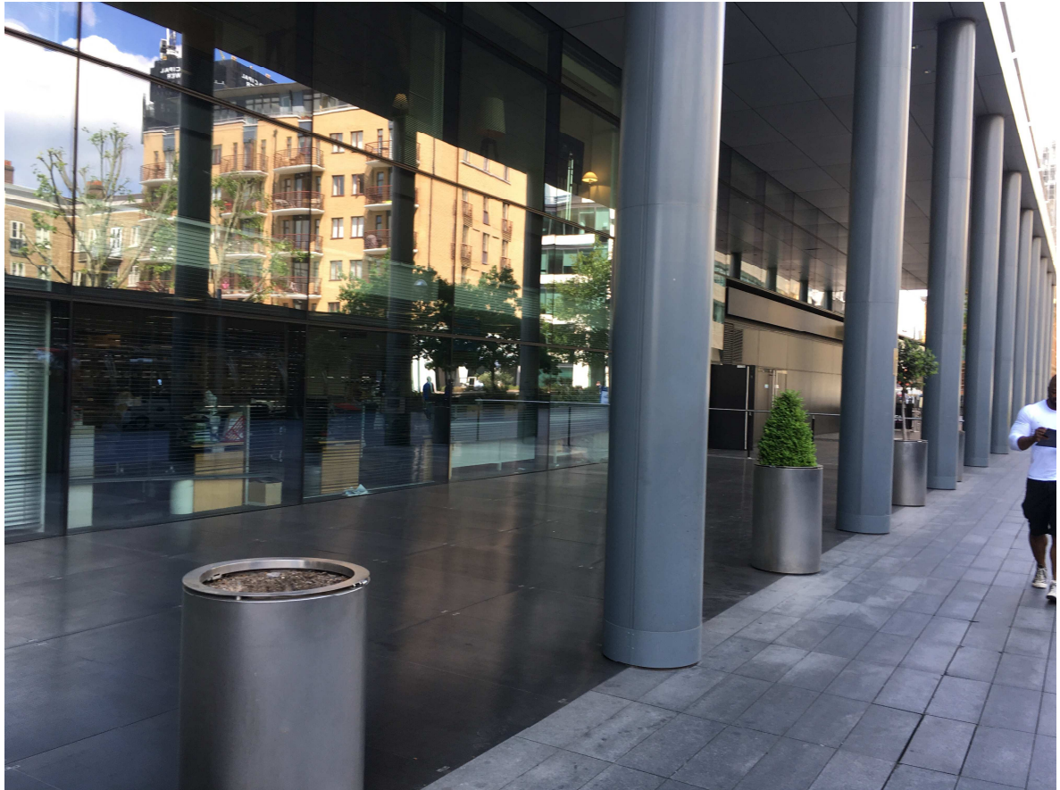
Image 5 - Lamb Street as existing (looking south-west)
